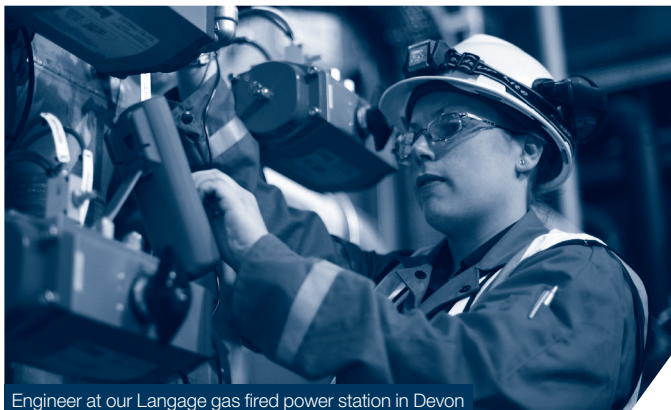
Engineer at our Llangage gas fired power station in Devon
