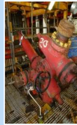
Fabric maintenance of 5 well-head Xmas trees
