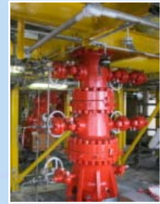
Fabric maintenance of 5 well-head Xmas trees
