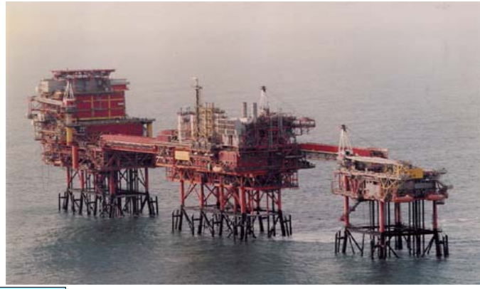
47/3B Installed 1983 24 wells 24/7 Operation
