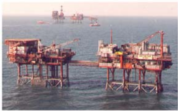
47/8A Installed 1977 6 wells 24/7 Operation
