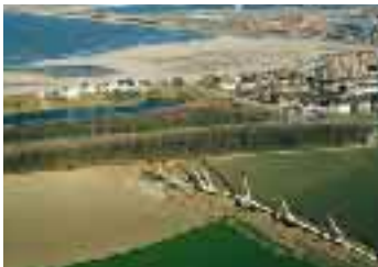
The new Interconnector gas pipeline gives Centrica access to Europe
